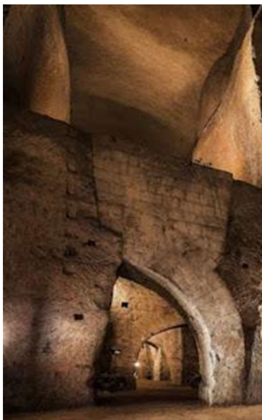
Figure 4: San Lorenzo Maggiore , a 13th century church in Naples, the foundations made of tuff stone.
