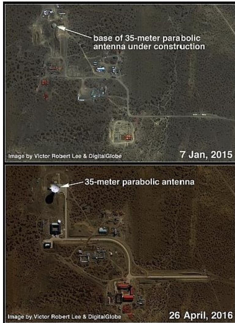
Figure 3: Space-Monitoring Chinese Base Project
