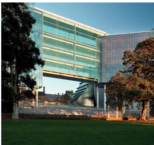
(Image of the site for the studio project: Public Park in the Foreground; Fence, Stairs and Law Building Beyond) (Francis-Jones Morehen Thorp Architects)
