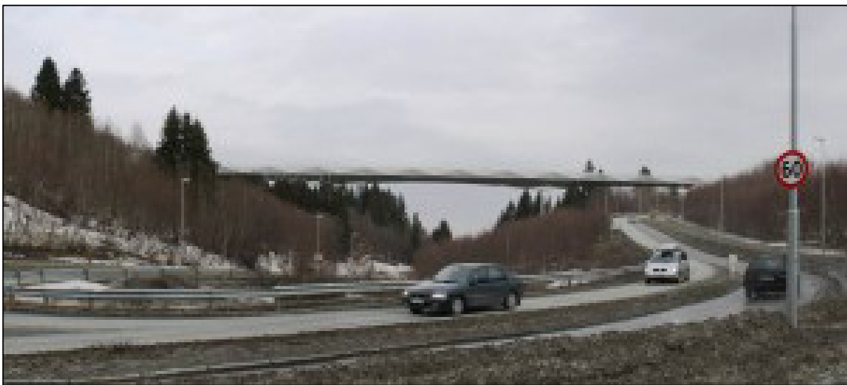
Figure 5: Picture (from the south) with a sketch of the bridge
